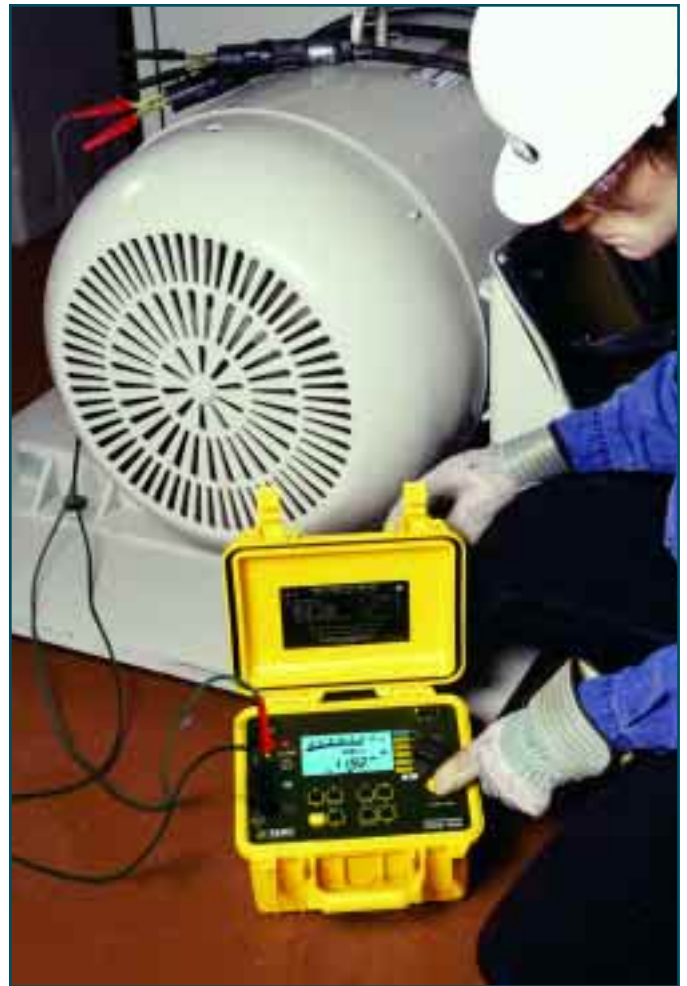
Model 5060 checking insulation resistance on feed cables to a 3-phase motor.
