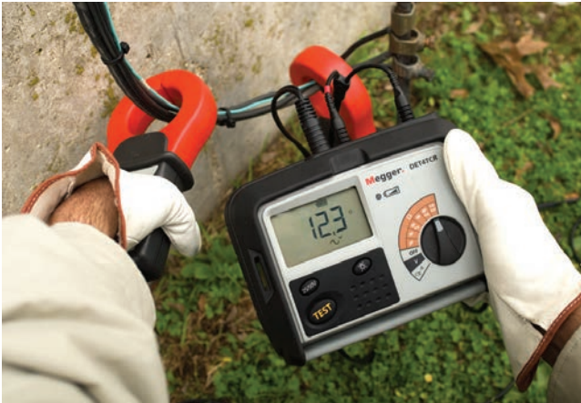
Model DET4TCR2 shown performing the stakeless ground testing method using only clamps.
